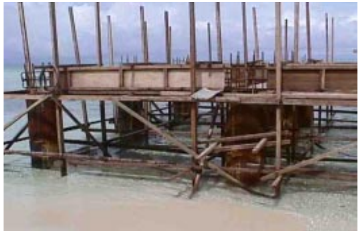
Status of new ranger station, December 1999
